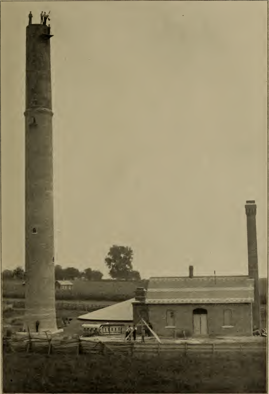
STAND TOWER—JERSEYVILLE, ILLINOIS.
